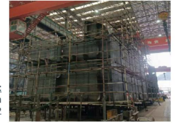
Right: Block Fabrication for Hull MW628-12
